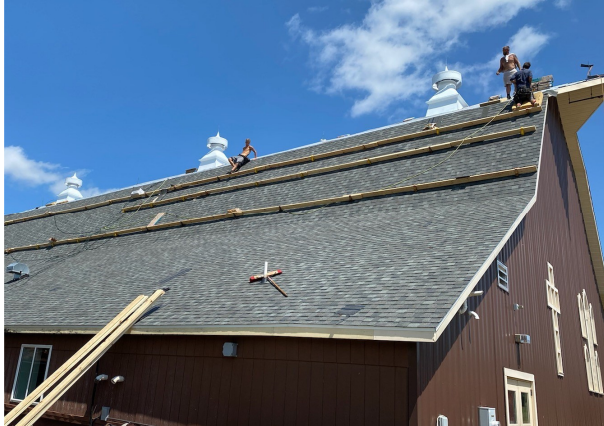
Reroofing the Chapel
